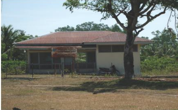
Port weigh bridge and office
